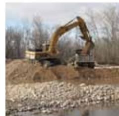
Gravel removal helps control water flow on the Boise River.
