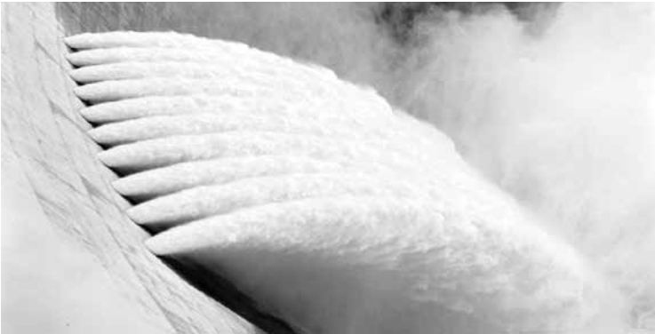
A row of cast-iron valves shoot water through Arrowrock Dam.
