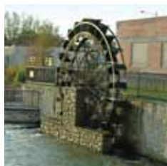
A functional water wheel is a prominent feature along Indian Creek.
