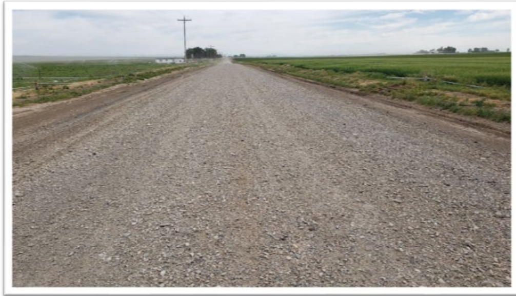
Picture 2.2 Finished Gravel Road
