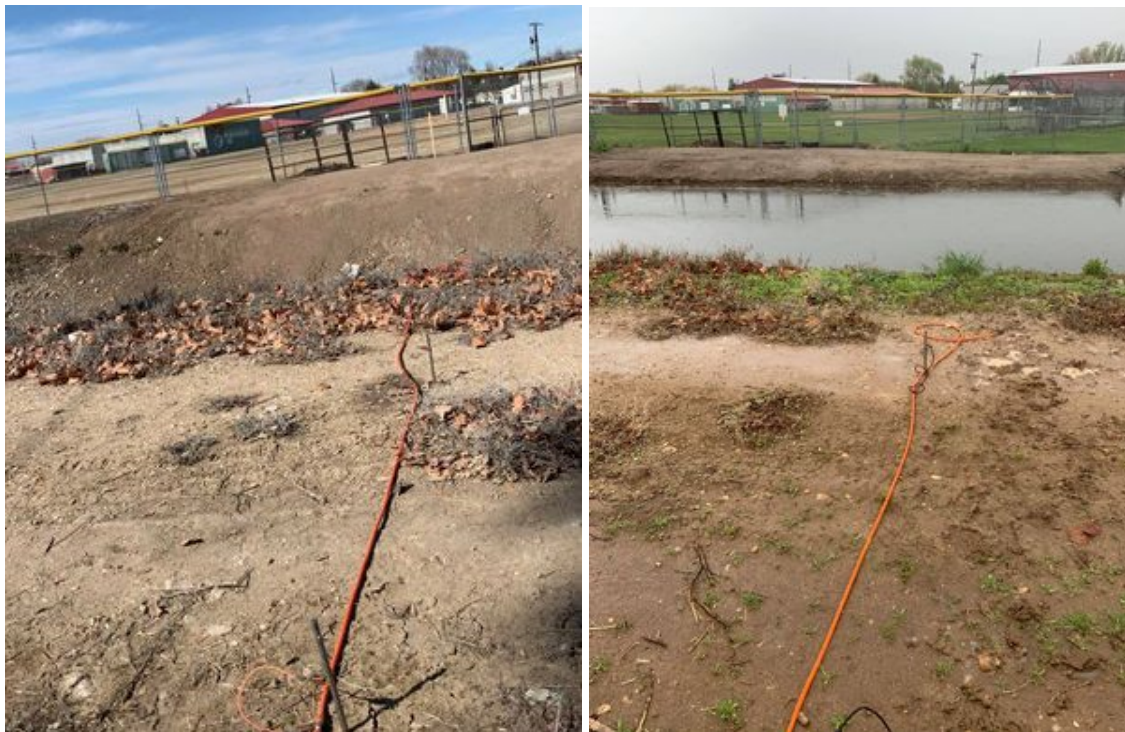
Photo 3.1 First electrode installed at approximately 1 m away from the canal edge
