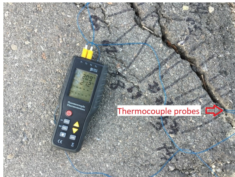
Figure 3- 7. Thermocouple is used for measuring the mean temperatures inside cracks
