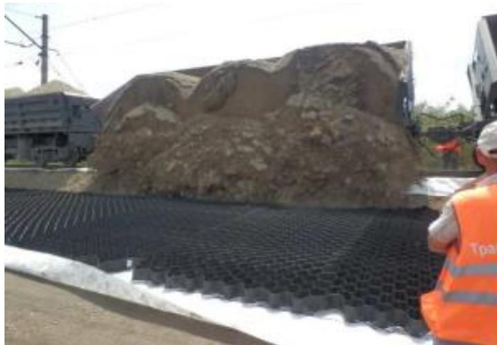
**Figure 2.9 Geocell-Geotextile Hybrid System**
