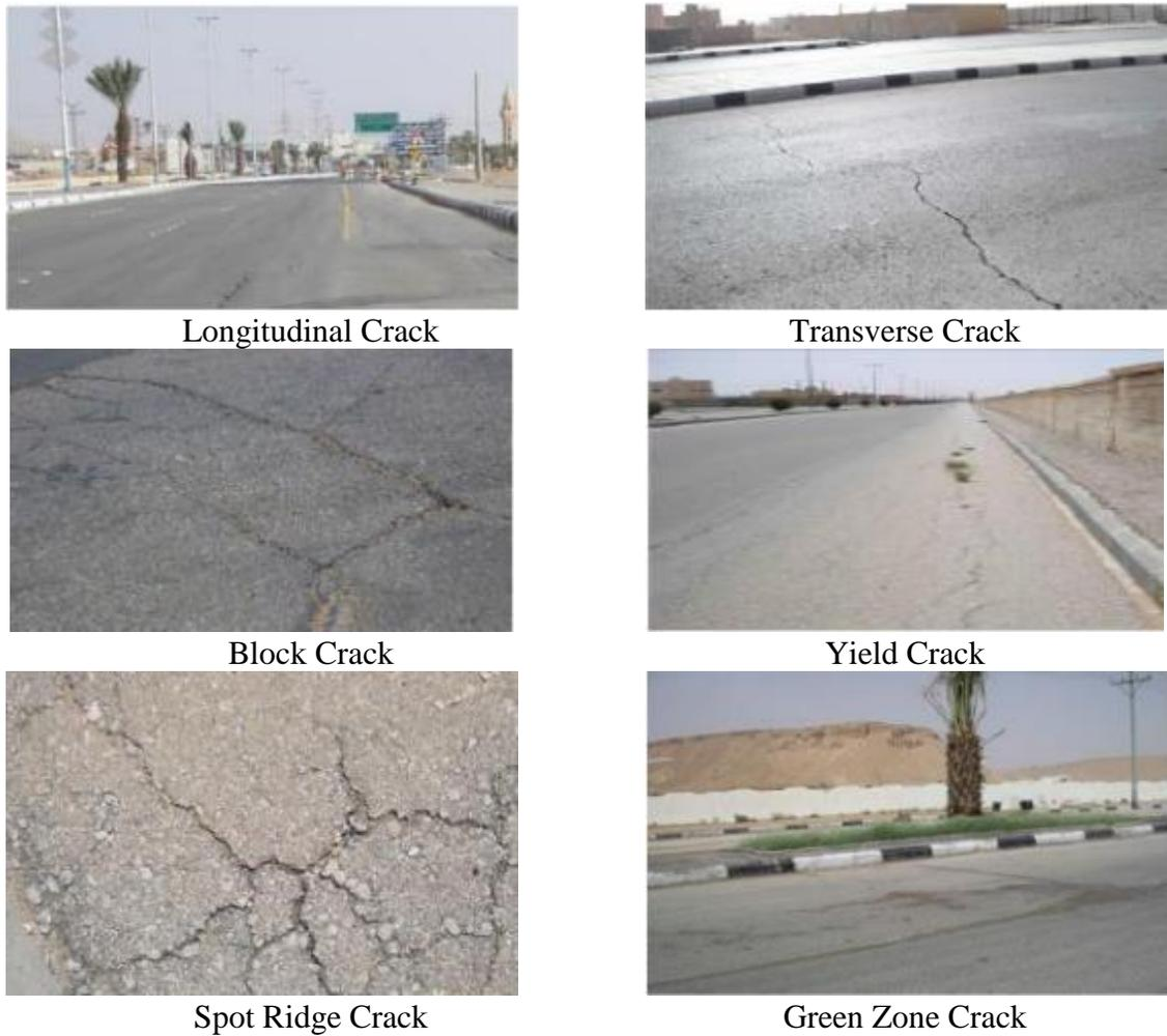
**Figure 2.2 Crack Types Associated with Expansive Soils (Dafalla and Shamrani 2011)**
