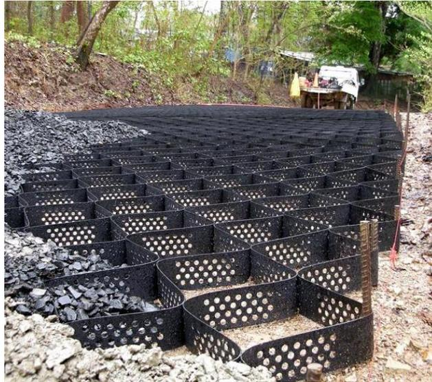
**Figure 2.5 Geocell Application in Roadway**
