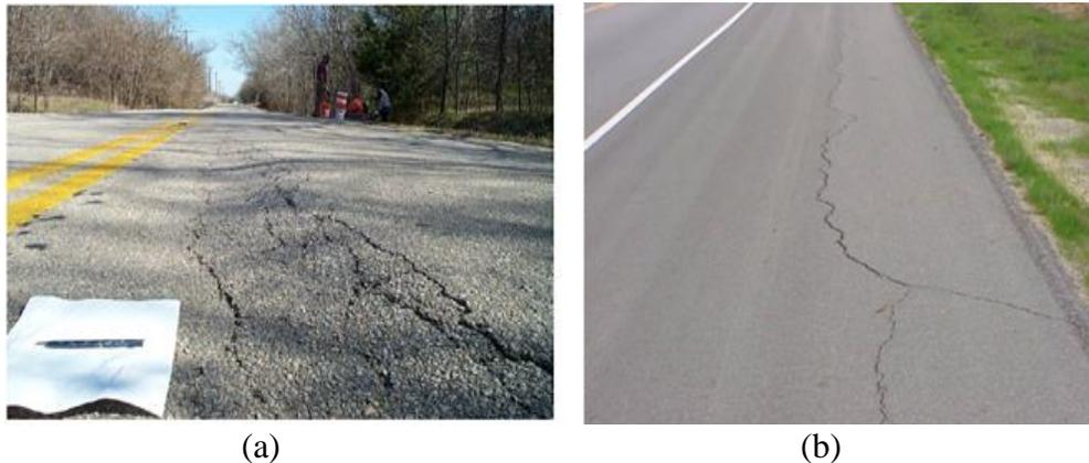
**Figure 1.1 Photographs Showing Damage to Pavement Systems due to Volume Change in Underlying Expansive Soil Deposits (Manosuthikij, 2008)**
