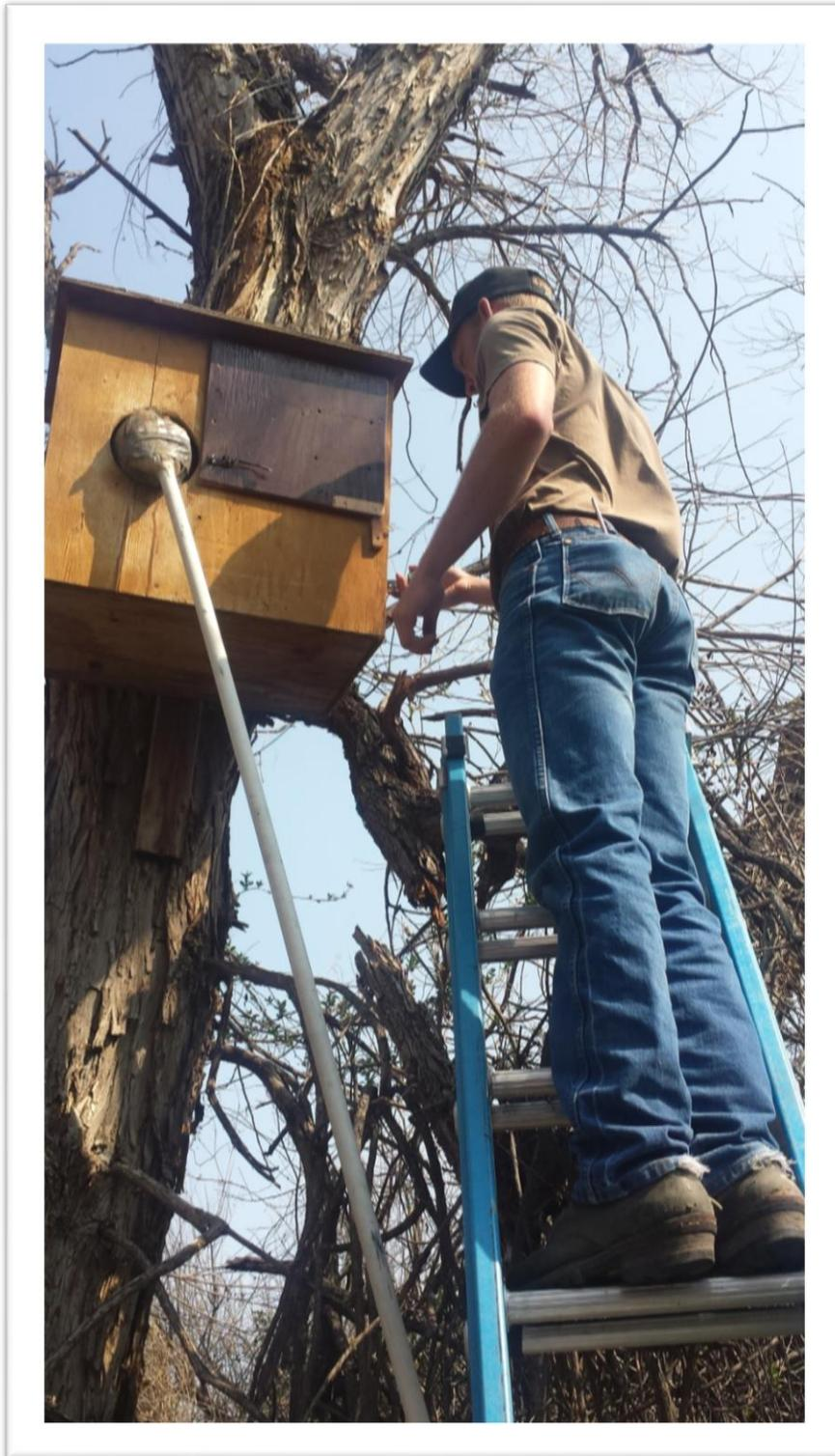
**Figure 3.5.** Installation of laser-break triggered trap door on a Barn Owl Nest Box near CJ Strike Reservoir, east of Grand View, Idaho, USA.
