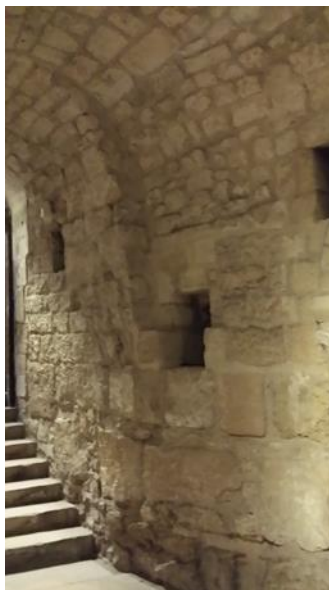
Figure 5 Fulrad's Apse and Stairs to Upper Nave of Twelfth Century Building. 163
