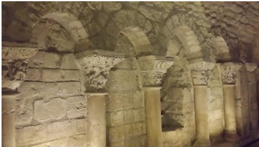
Figure 34 Exterior of Fulrad's Chapel Inside Suger's Crypt Ambulatory. 357
