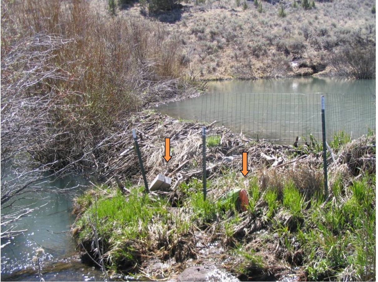
Figure 26. The remains of the irrigation dam (orange arrows). Originally built to encourage beaver settlement, the irrigation dam became barely visible underneath repairs made by reintroduced beaver. This picture was taken in 2007, six years after the reintroduction of five beavers at the dam site.
