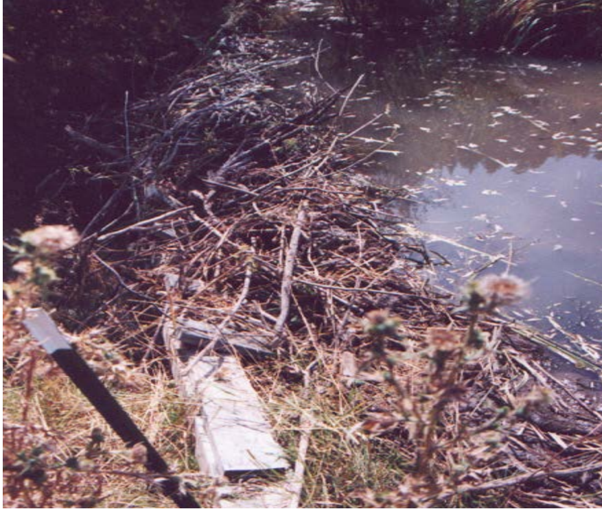
Figure 22. Repairs made to the irrigation dam by newly-resident beaver during the summer months of 2002. Five beaver were reintroduced, during August and September of 2001. The irrigation dam was designed to preserve spotted frog habitat in the reservoir above, and to encourage settlement by beaver released at the site.
