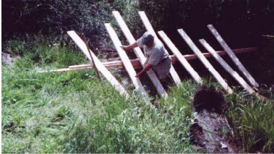
Figure 17. Framework of the irrigation dam built in 2001. The dam was designed to slow the flow of Stoneman Creek in order to provide suitable spotted frog habitat and to encourage settlement by beaver that were released into the reservoir following repairs.
