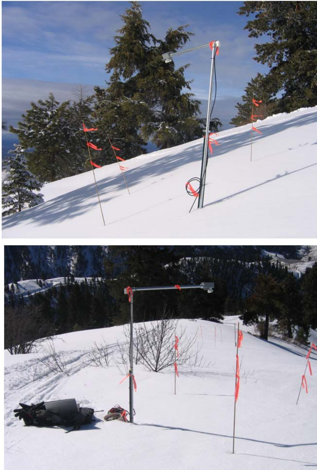
Figure 10 USD sensors and data acquisition at Lower Deer Point site
