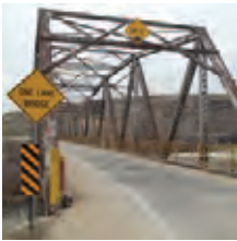
BRIDGE AT CANYON CROSSING
