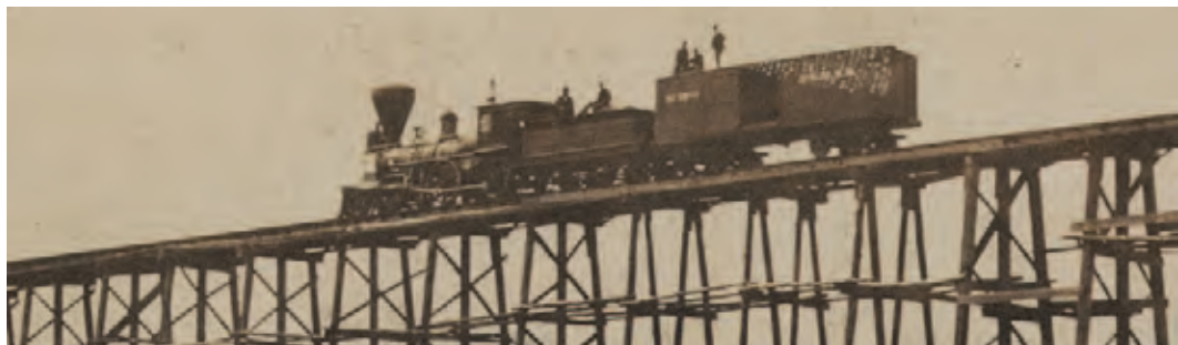
Wooden trestles bridged Idaho's fractured landscapes.
