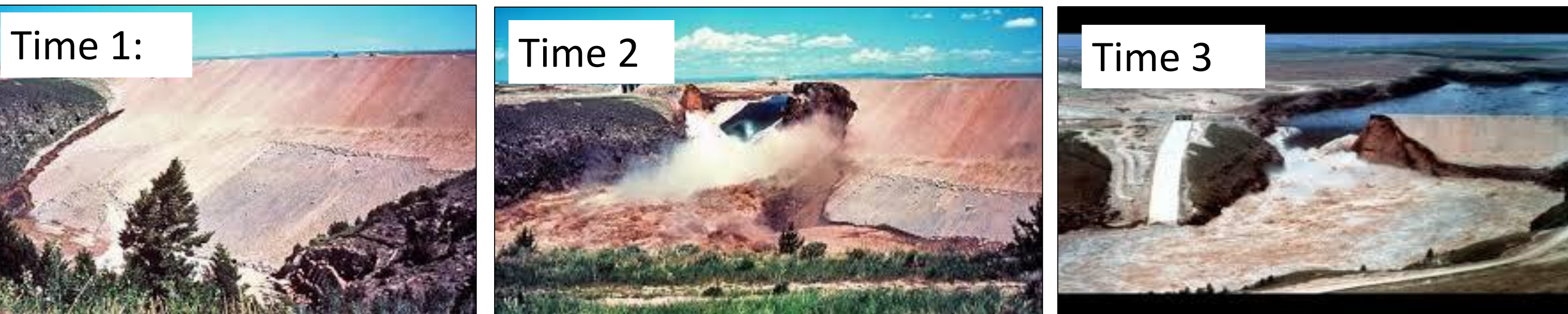
(Above) The historic Teton Dam Failure. Left picture: 11:52 AM. Right picture: 11:58 AM. (Bureau of Reclamation).
