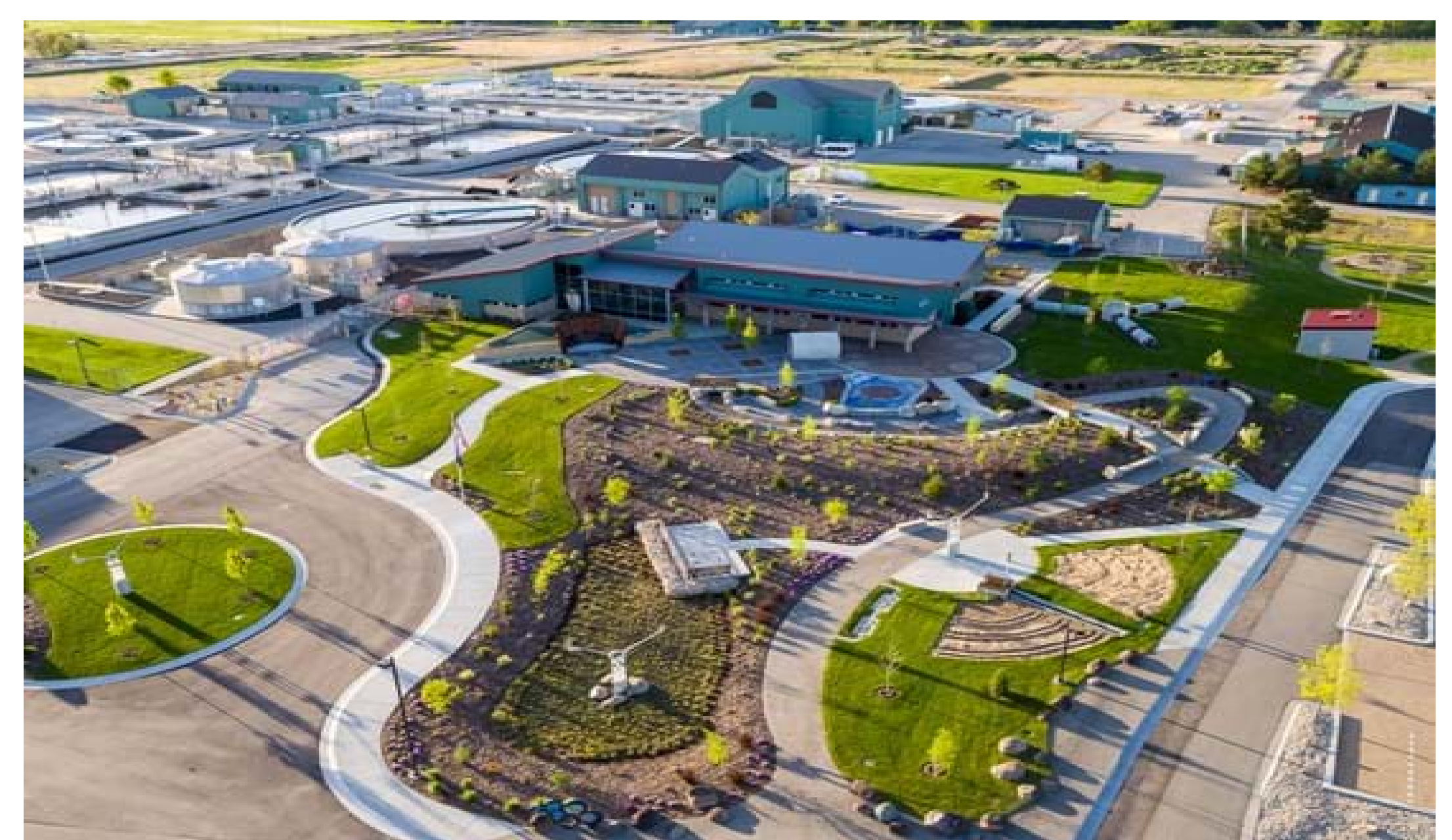
FIG. 1: Boise WaterShed outdoor facility; Boise, ID.
