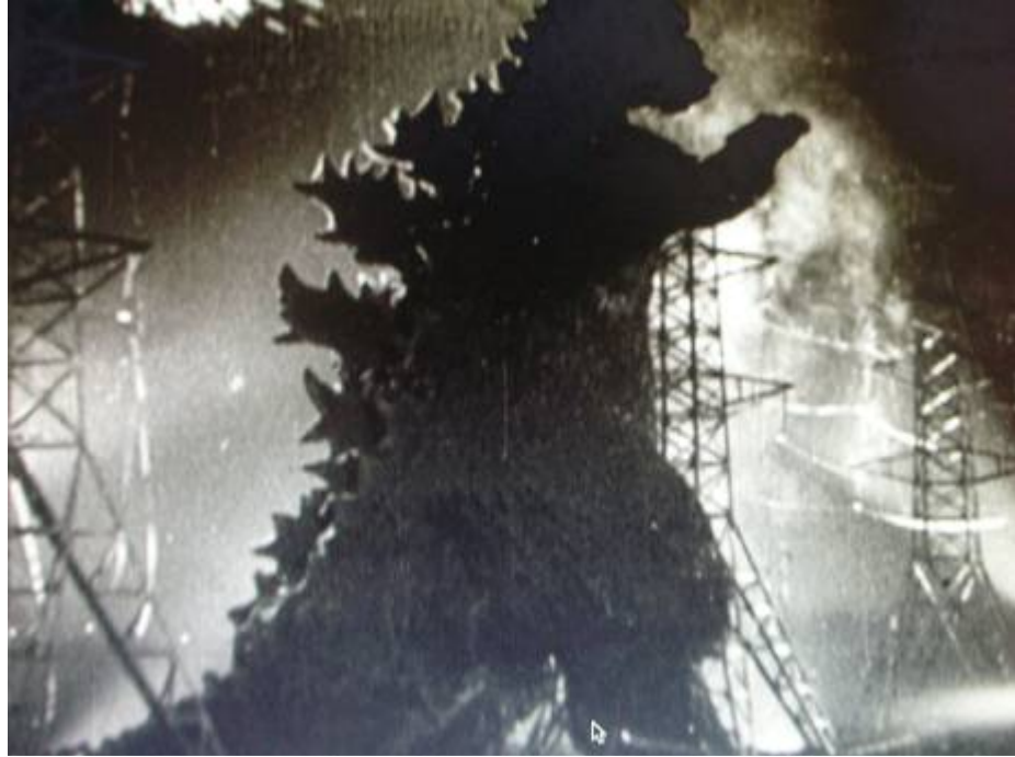
Figure 7. Gojira lays waste to Tokyo
