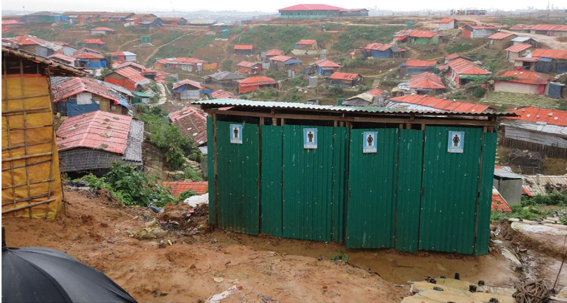
Figure 5. Four toilets built on a steep slope serving those living in surrounding temporary shelters.
