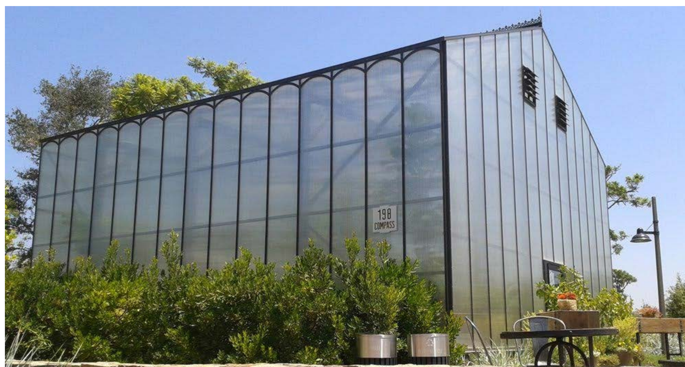
Five-wall insulated polycarbonate greenhouse from Gothic Arch Greenhouses similar to one needed for IPC.
