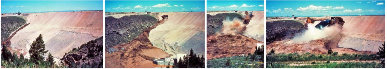
Figure 1.2: The historic Teton Dam Failure documented by the Bureau of Reclamation photos occurring at (A) 11:30, (B) 11:40, (C) 11:57, (D) 12:05 occurring on 5 June 1976 (Reclamation, 1976).
