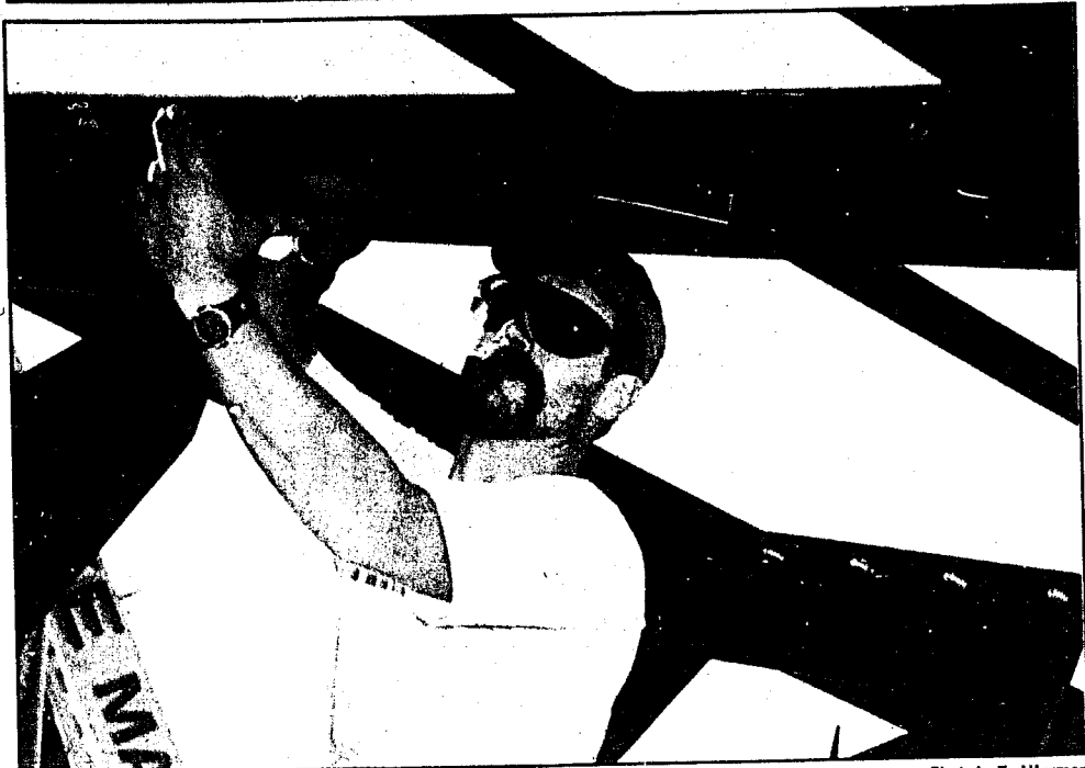
Dan Chaudoin of Yanke Machine Shop tightens up one of the final bolts on the new kiosk along the sidewalk outside the SUB. The individual pieces of the structure were manufactured in the shop and then assembled on-site.
