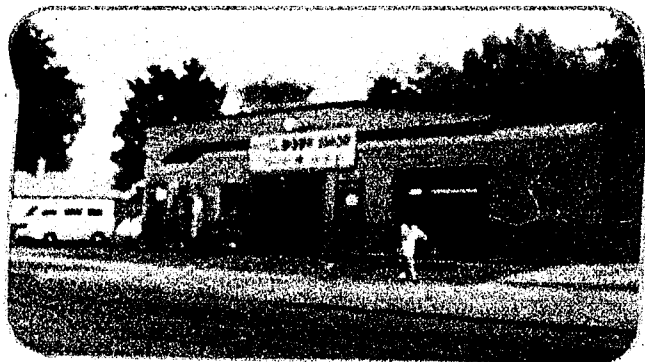
The auto body shop on University will be demolished to make room for the rec center
