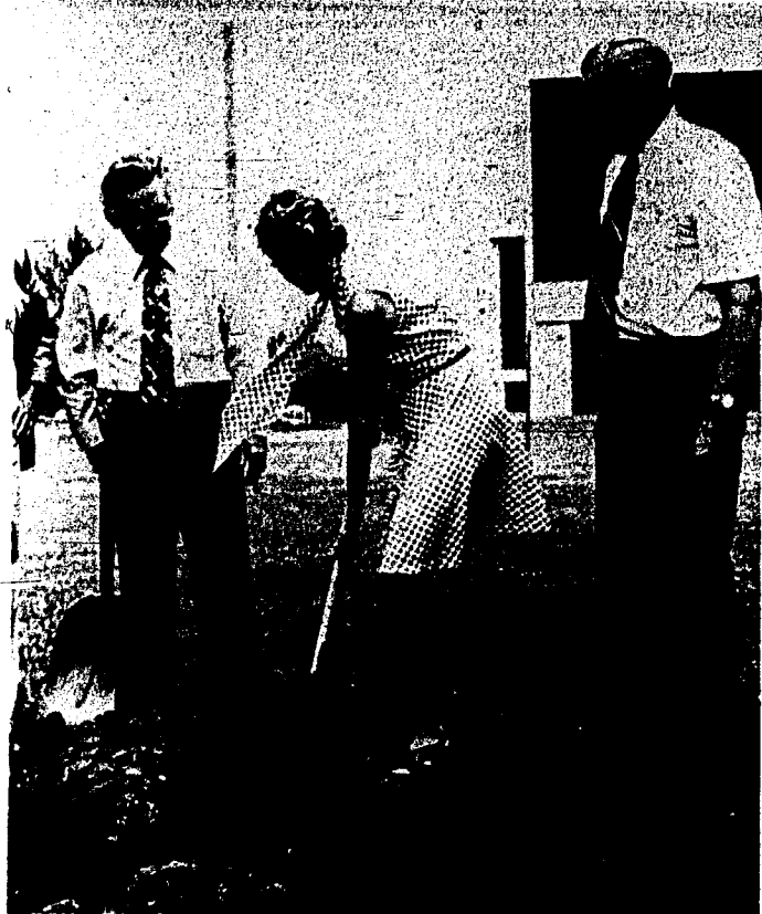
The ground breaking for the new Science-Education building was held in July. The construction is expected to be complete the early part of 1978.
