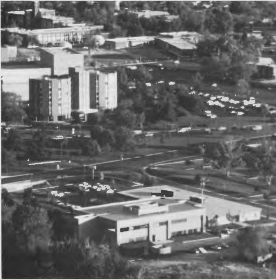
Boise State has agreed to purchase two classroom buildings (foreground) that now house the ITT Technical Institute. But the university won't use the space until the institute's lease expires in 1995.
