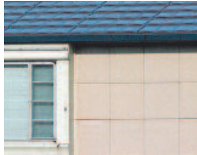
Lustrom of Ohio prefabricated a powder-blue porcelain-enameled steel ranch-style house for the postwar boom, 1947. Opposite: the Detrioter advertised a pre-furnished maintenance-free home, 1959.
