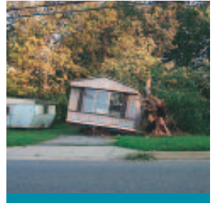
Wind damage, Maryland. Opposite: Martin's Mobile Village, Redmond, Washington.
