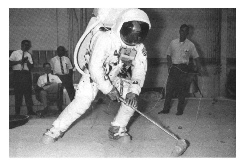
to accomplish the task of collecting different lunar samples. A collection of tongs, rakes, scoops and collection bags were used to obtain rock samples ranging from tiny pebbles to inch sized rocks.
